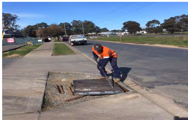
Removing pit lid
