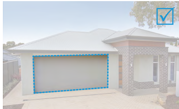
Figure 19 Garage should be recessed and not a prominent feature of the building.
