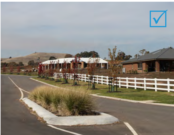
Figure 12 Low level planting allows for clear sight lines at vehicle exit points.
