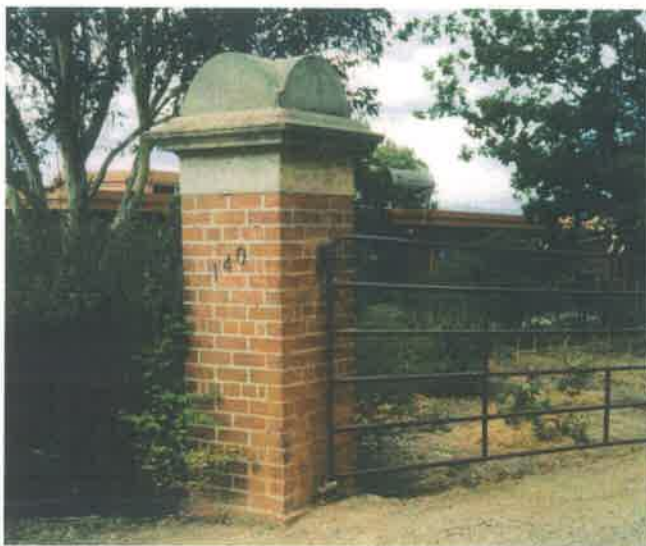
Existing front gate
