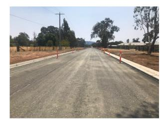
The construction and sealing of 550m of Withers Lane has commenced. Kerb and channel and drainage works have been completed in the first section. Works are expected to be completed in early February 2020.
