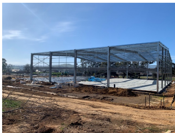
View of Sports Stadium Structure
