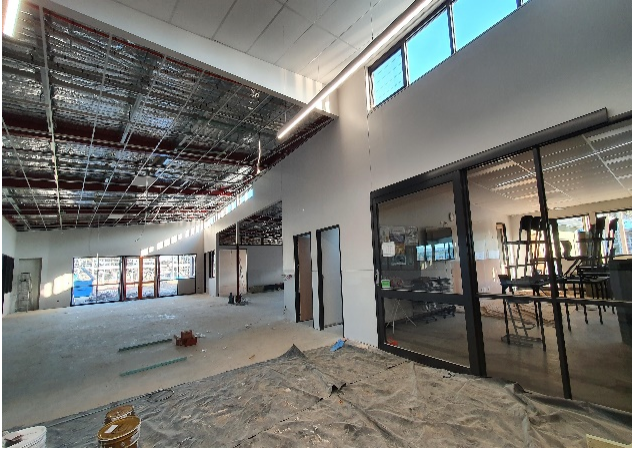
Internal View of STEM Building
