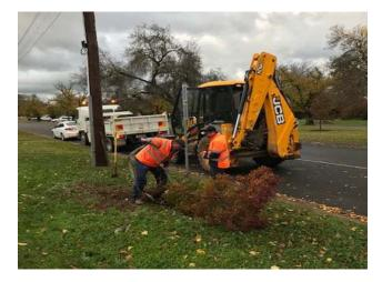
Maintenance works have been completed on the Mansfield Township High Street centre median strip. The soil in this area has been somewhat lacking due to foot traffic and compaction. The soil has been aerated to aid better water penetration and root formation of trees, this should also improve the grass areas.
