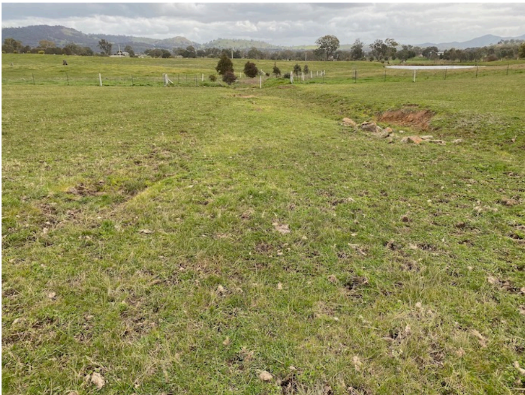
Figure 6 – Small amount of gully instability
