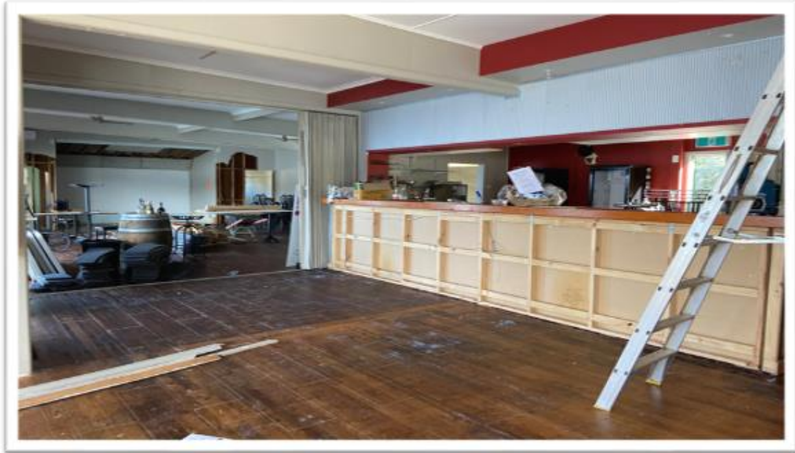
Bar and Dining Area During Strip-out
