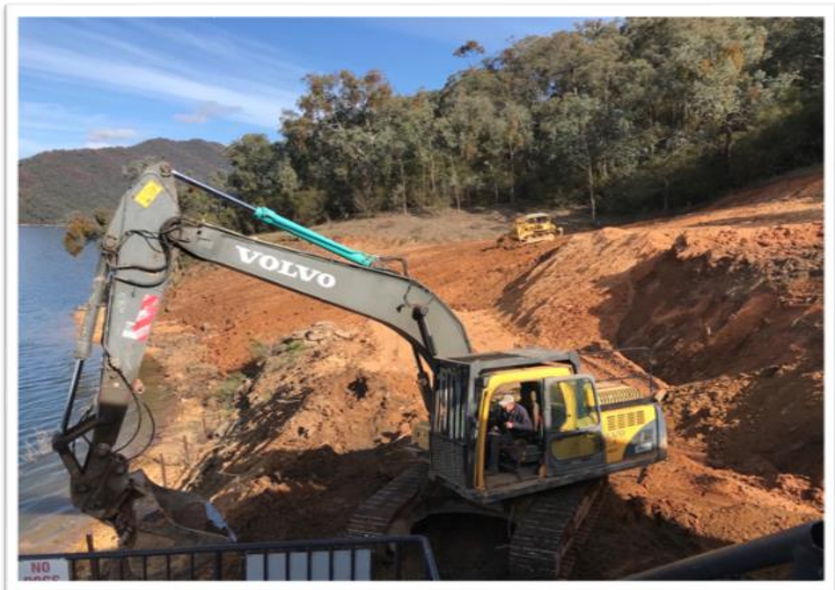
Excavation to extend south car park and access road
