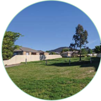
Figure 2.1: Mitchell Court Drainage Reserve
