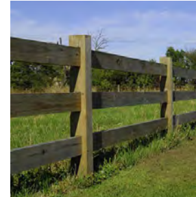
D. boundary fence along Monkey Gully Road
