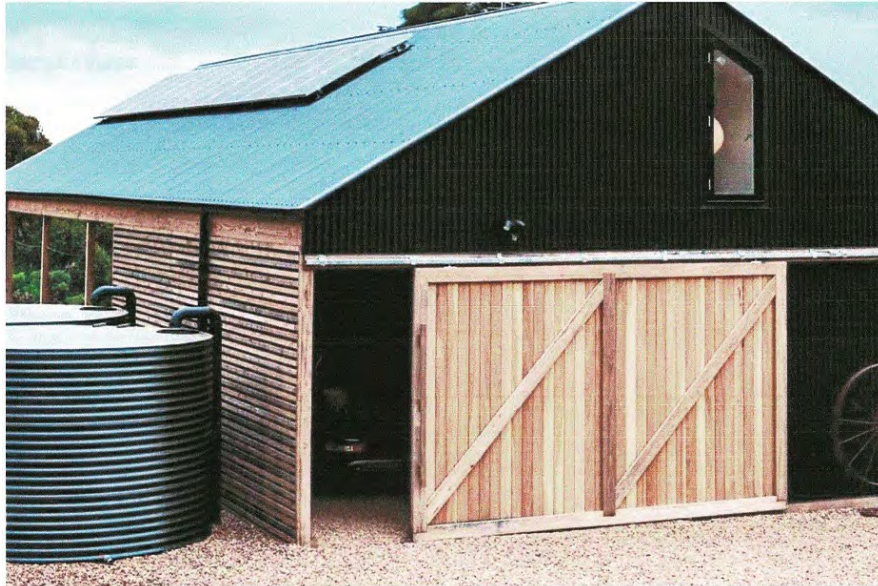
Image: Metal shed with timber siding on ends and doors
