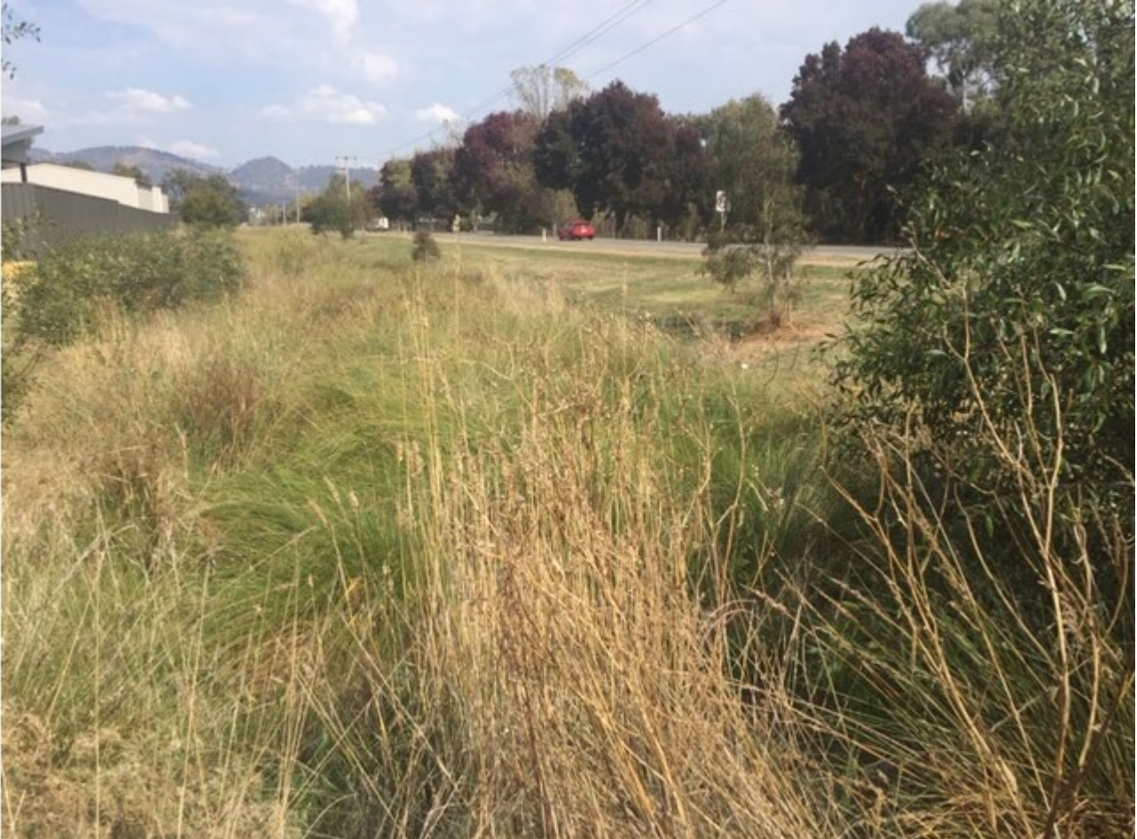
Figure 2 - Bio-retention swale running along-side the Mansfield-Whitfield Road that is subject of the bond
