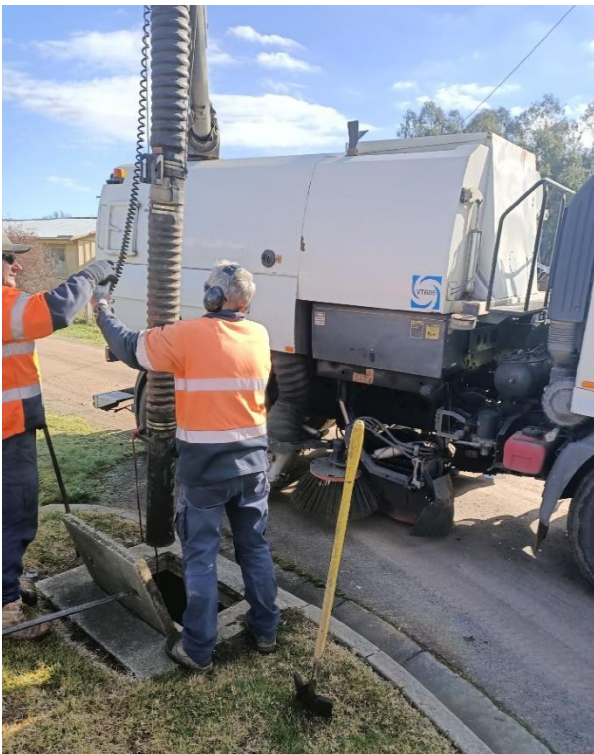
Street sweeping truck overhead suction boom being used to clean stormwater pits, and kerb sweeping reducing manual handling significantly for outdoor staff.
