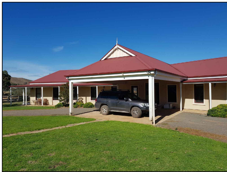
EXISTING HOUSE FINISHES
