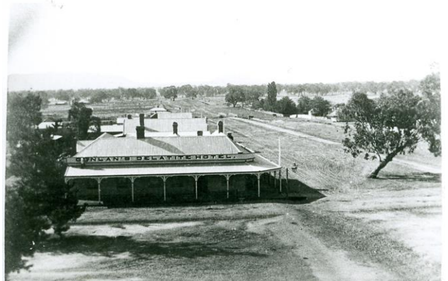
Delatite Hotel in its single storey state (MHS Photograph No.6)
