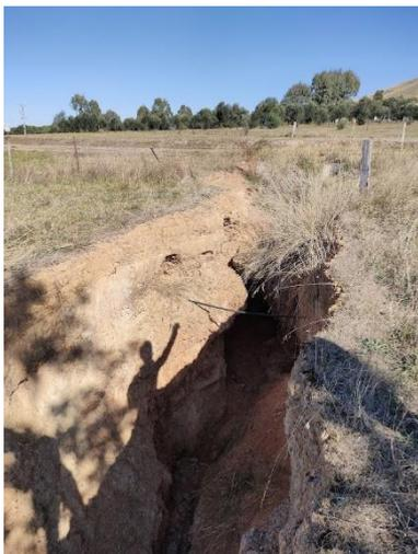
Historically road drainage enter the property at this point. This gully is approximately five meters in depth. While this historical damage and a majority of the water has been diverted, yet water still flows through this gully.
